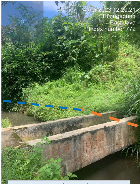
Jembatan Pipa (crossing) Talang Air
